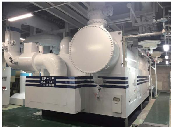
Photo: The recently installed 5,400 RT inverter turbo chiller
