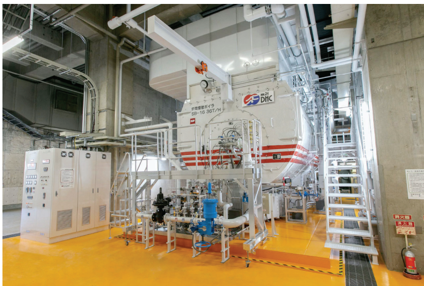
Flue and Smoke Tube Boiler
